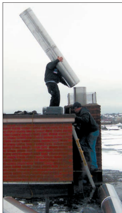
A rigid liner being assembled.
