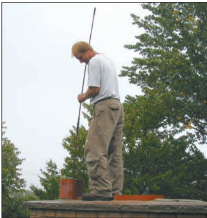
The chimney should be cleaned thoroughly before relining.
