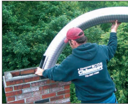
Flex liners are the most common type, and must be used for relining chimneys with offsets.
