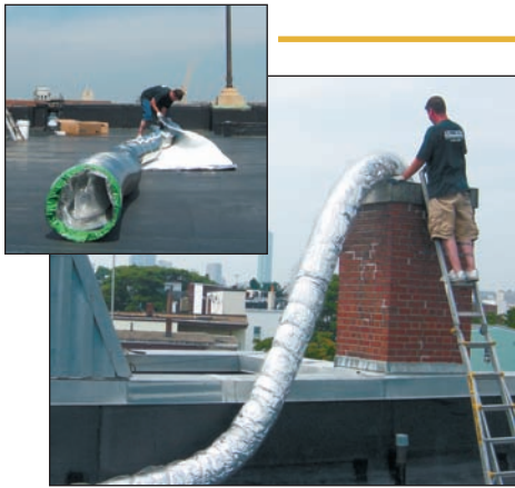
Blanket insulation must be carefully installed.
