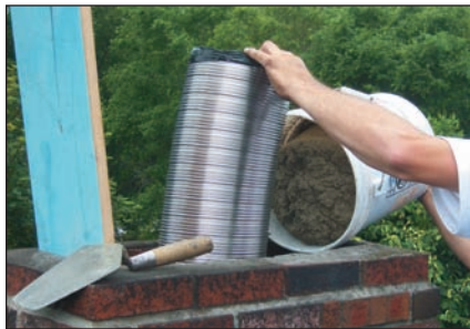
Installing mixed insulation around the liner.
